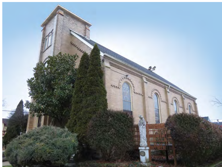
Church: 140 West Avenue
