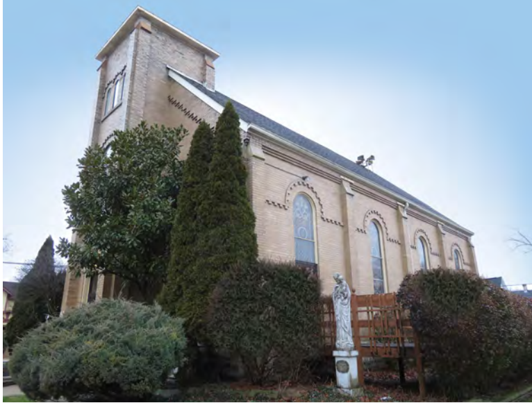
Church: 140 West Avenue
